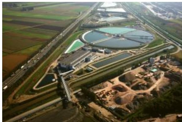
AMORAS sludge treatment plant ( www.amoras.be/en/project )
